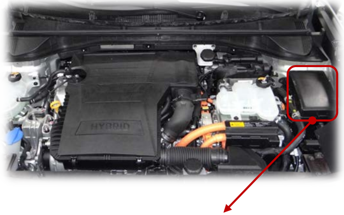
Engine room fuse box
