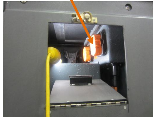
Master Service Disconnects
